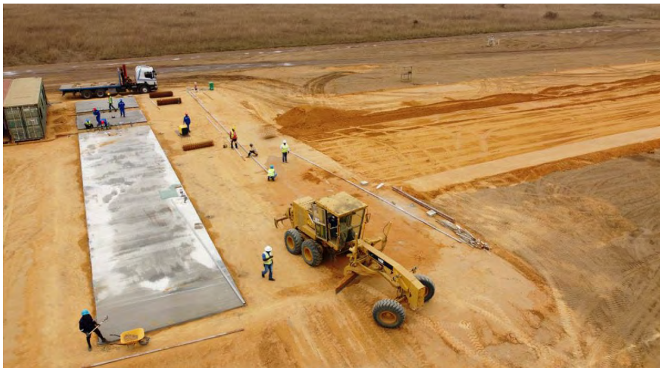
Figure 25: Aerial Photo of the Construction Camp. Mobilization area - raft slab. Water Supply Management (OEC photo)
